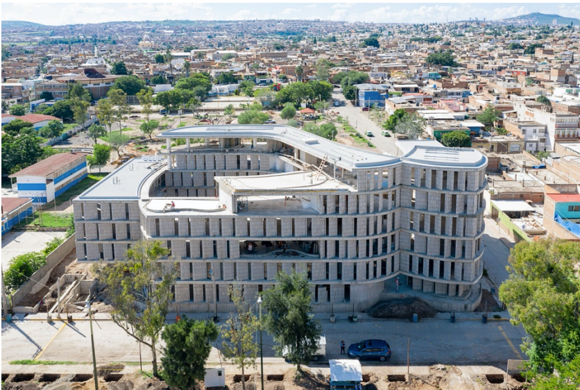
In León, Mexico, the Las Americas Social Housing Project comprises 60 condo units, arranged vertically around a central courtyard so that no two apartments face each other. Iwan Baan
