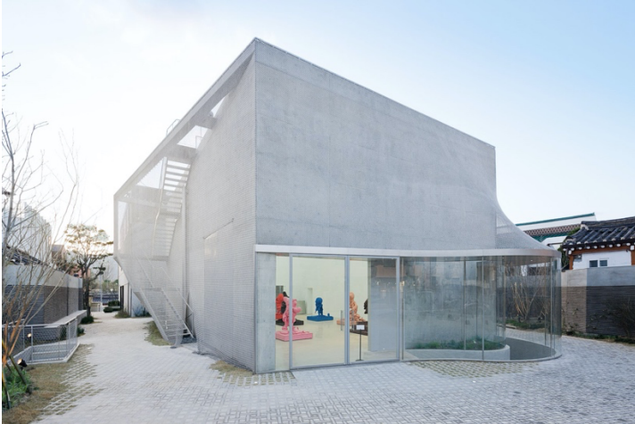
A chain-mail skin of some 510,000 interlocking metal rings cloaks Kukje Gallery in Seoul, one of the firm’s early successes. Iwan Baan
