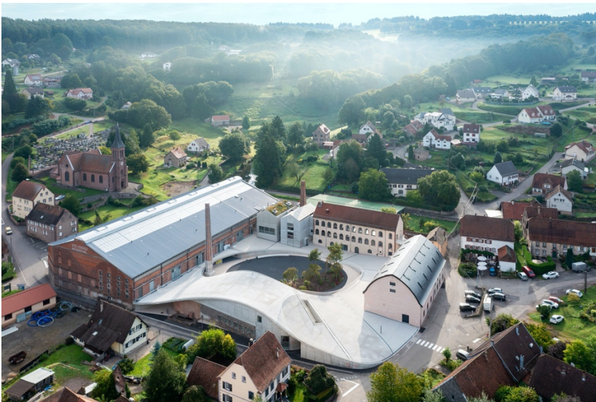
In the historic studio-glass center of Meisenthal, France, SO-IL united three neighboring institutions using an undulating concrete addition that frames a public plaza. Iwan Baan
