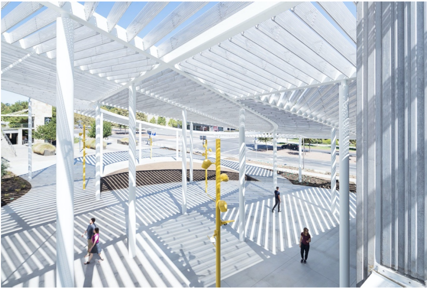
A canopy of aluminum beams extends over the site and the museum, which was conceived as a permeable forum for public engagement. Iwan Baan
